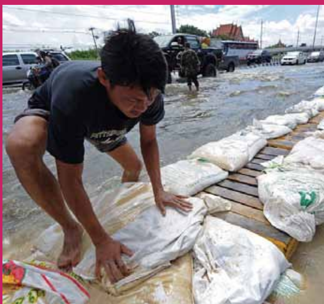
Flood defences protecting Bangkok, Thailand
