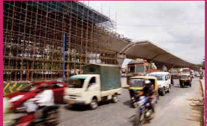
Airport road in Bangalore
